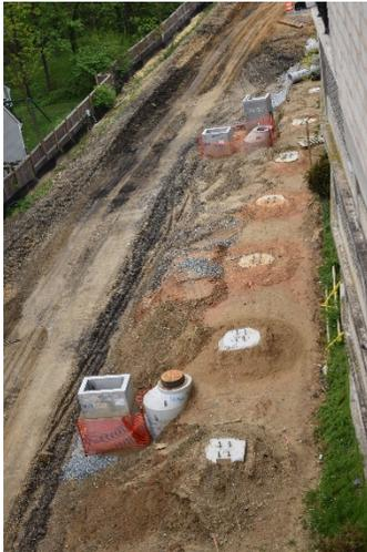
Response: These are noise wall footings. The exposed steel shown are anchor bolts for the steel posts.
