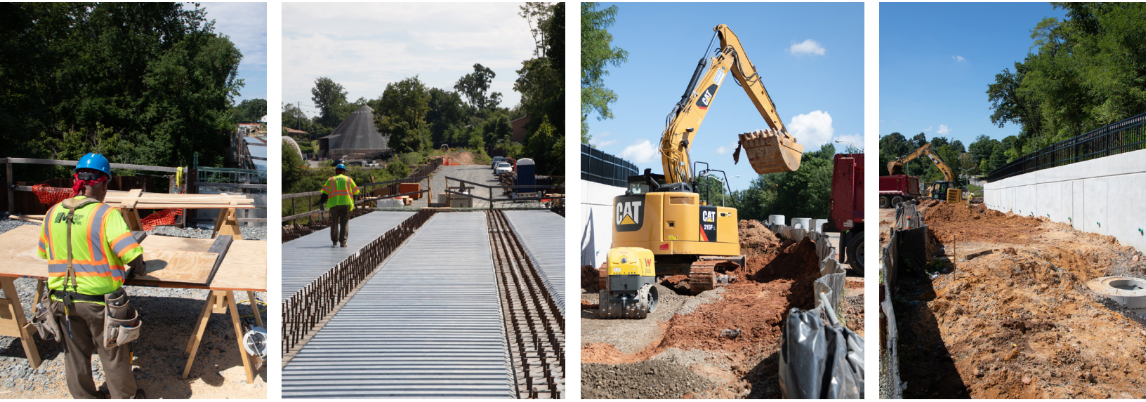
From left to right: Crews continue to advance construction of the light rail vehicle bridge over Rock Creek in Montgomery County. They are building the formwork for the bridge deck that will soon be filled with concrete. In New Carrollton, stormwater pipe installation continues in Prince George's County.
