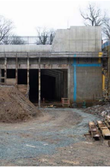
From left to right: Temporary supports are being removed to make room for the Wayne Avenue entrance to the future Manchester Place Station. Crews embedded track and cleaned the paint shop walls at the Purple Line OMF (Operation Maintenance Facility) in Lanham recently. Twenty-eight light rail vehicles will use the OMF as home base.
