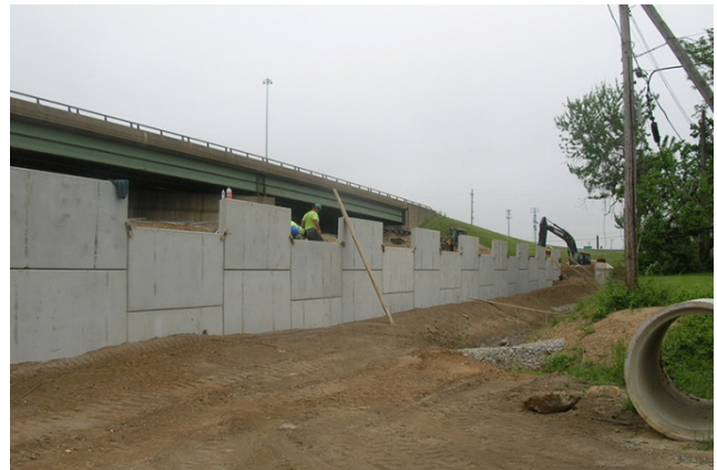
Figure 5-5. MSE Retaining Wall Construction
