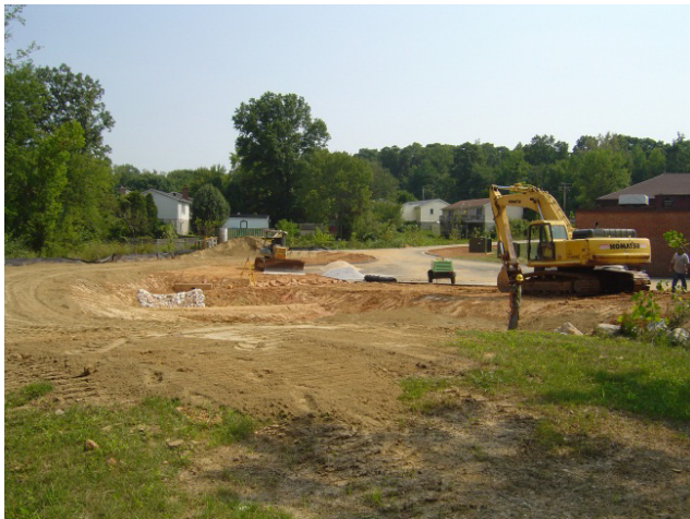
Figure 5-3. Examples of Site Grading and Equipment
