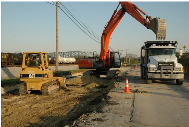
Figure 5-4. Example of Road Cut for Track Installation
