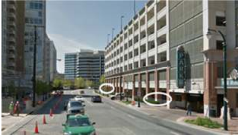
Photo #13: Wayne Ave Garage
