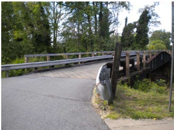
The existing structure has severe structural deficiencies which include inadequate load-carrying capacity and areas of section loss in the main load-carrying members. Load rating calculations for this structure indicate that legal vehicle loads in Maryland exceed the carrying capacity of the bridge, as it is currently posted for a 10,000 pound gross weight limit.
